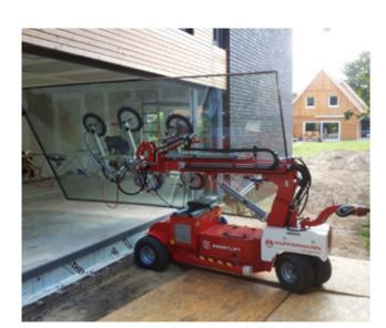
3D glass manipulators such as the radio-controlled and electric Sky Lifter from Smartlift work without any restrictions on working height. The machine – or loader crane – to which the glass manipulator is attached, is used as a glass installation crane. The vacuum suction cups are telescopic, enabling both exterior and interior glazing. Hydraulic operation is precisely controlled by radio remote control.
